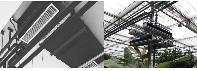
ULTRA-THIN, CEILING CONCEALED TYPE FCUS, SUITABLE FOR HOT/CHILLED WATER SYSTEM.
